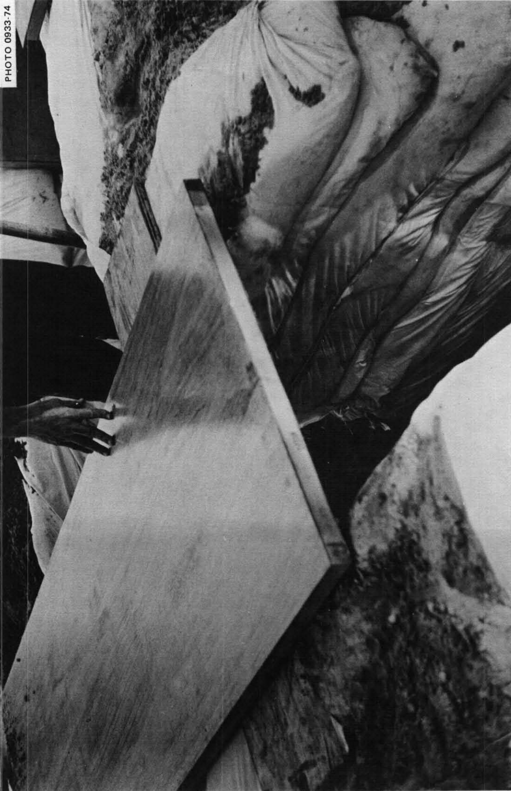
Fig. 5.8. Placing an interior door over one end of the shelter and part of an entryway. The wall of this entryway consisted of 7 small rolls which were made by using pieces of sheets and other cloth, with the outer ends tucked in. The man was standing on the main part of the shelter, over which other doors were soon to be placed, all parallel to the pictured door.
